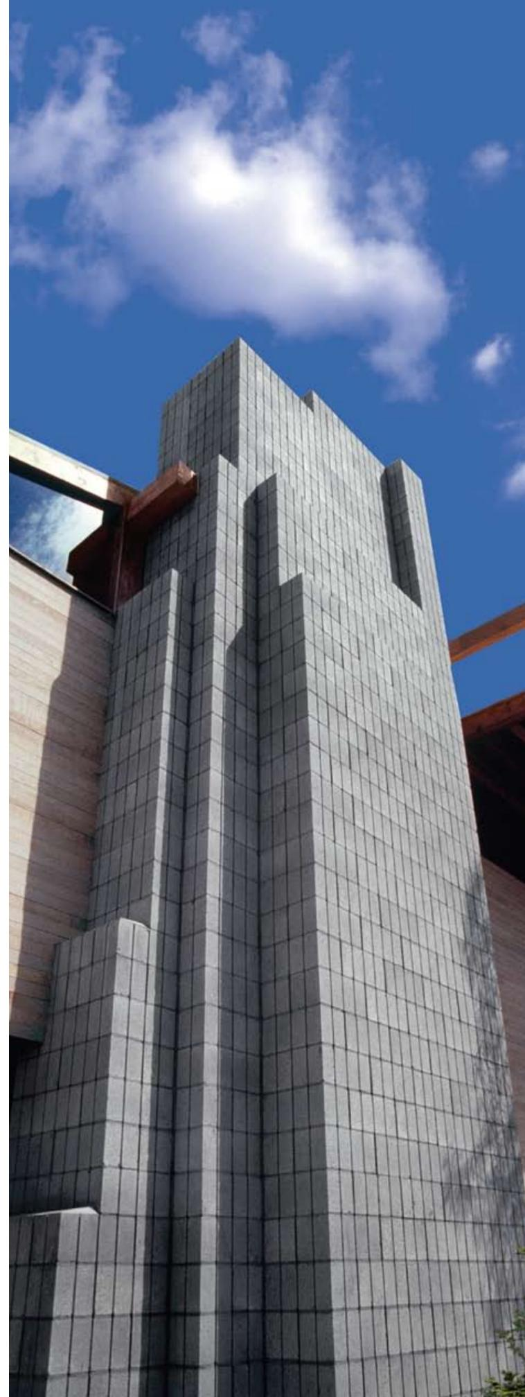
LEFT: What appears to be a skyscraper is really a chimney that scales one side of the home rising up 25 feet. An Applebaum innovation, exposed concrete blocks stacked with reinforced steel allow the structure to cantilever back into the chimney mass for seismic stability of the architecture.
